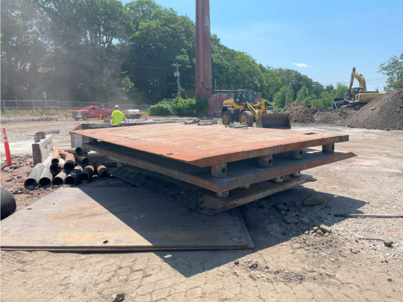
Photo 1. Trench Box removed from site observed.
