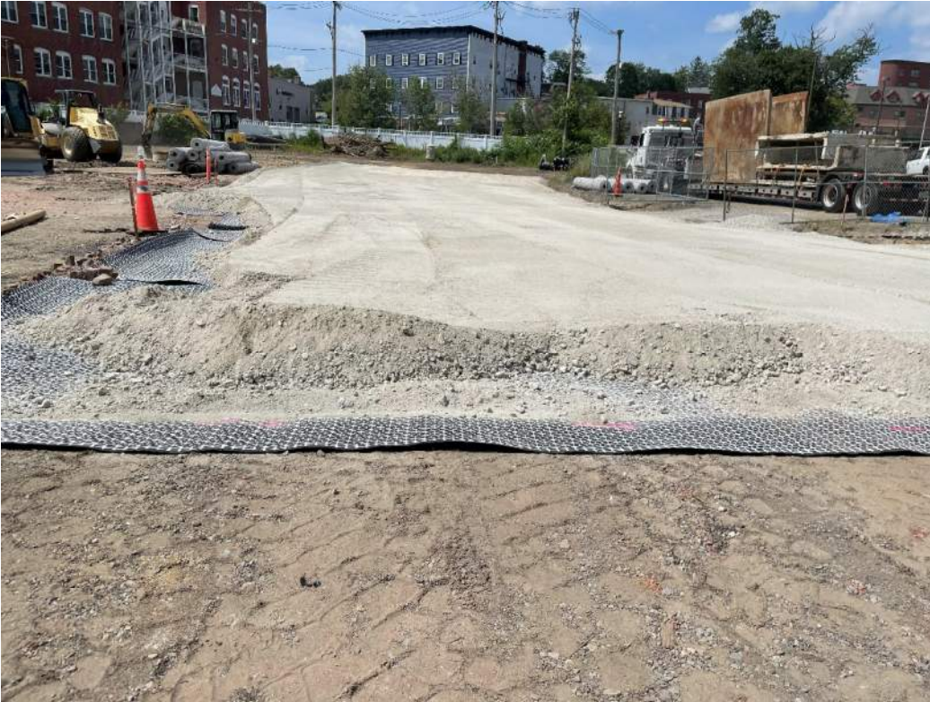
Photo 3. Eastern section of modified subbase installment.
