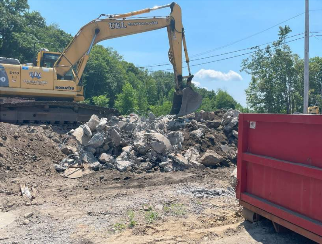
Photo 2. Large excavator observed removal of boulders and wire materials.
