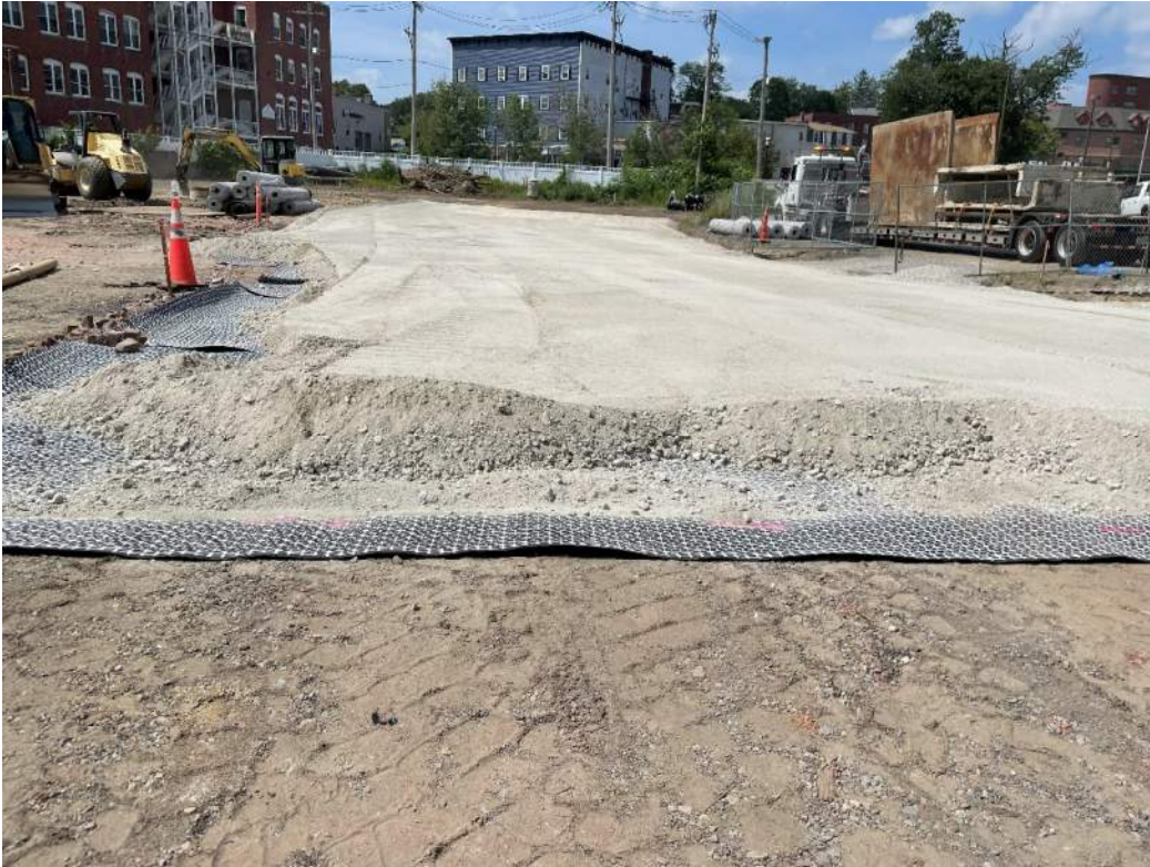
Photo 3. Eastern section of modified subbase installment.
