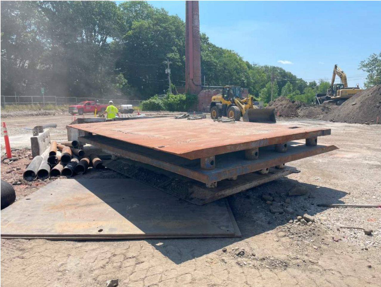
Photo 1. Trench Box removed from site observed.
