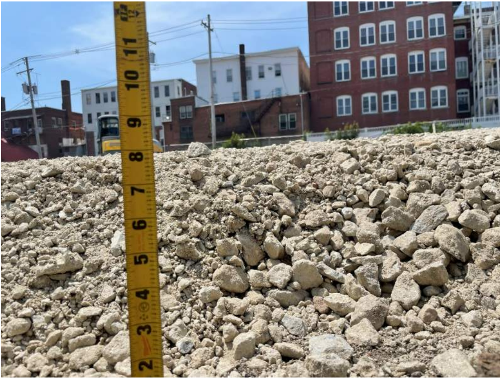
Photo 4. Compacted processed gravel subgrade at 8 inches.
