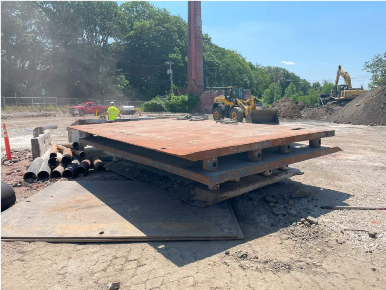
Photo 1. Trench Box removed from site observed.
