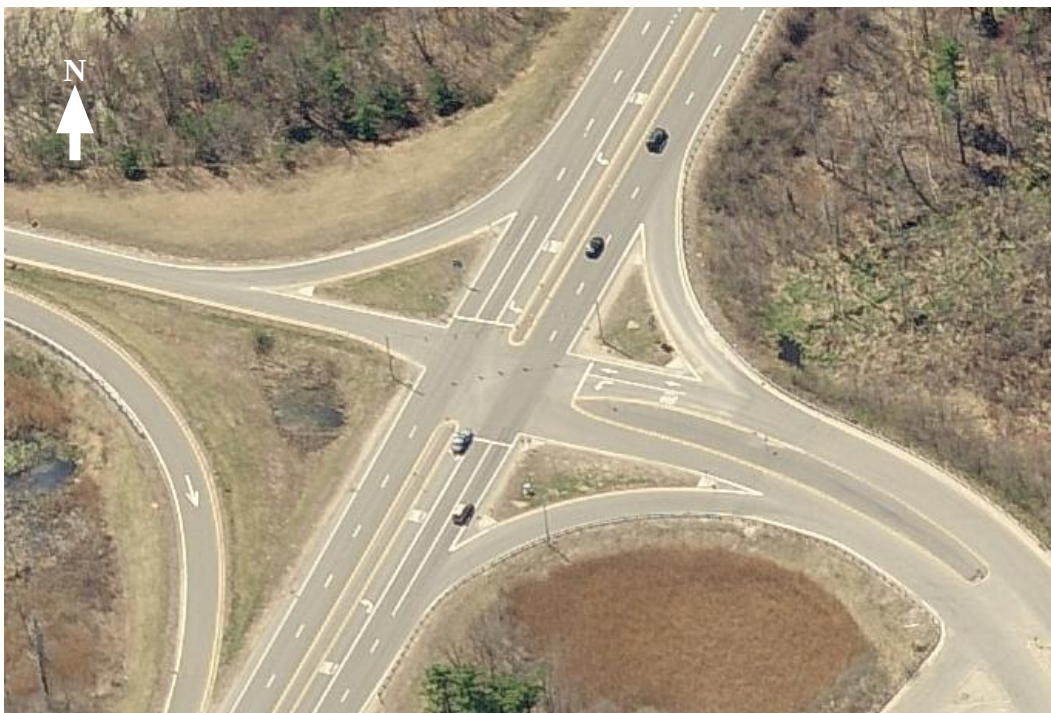
Route 140 at Simplex Drive/Route 2 Westbound Ramp
